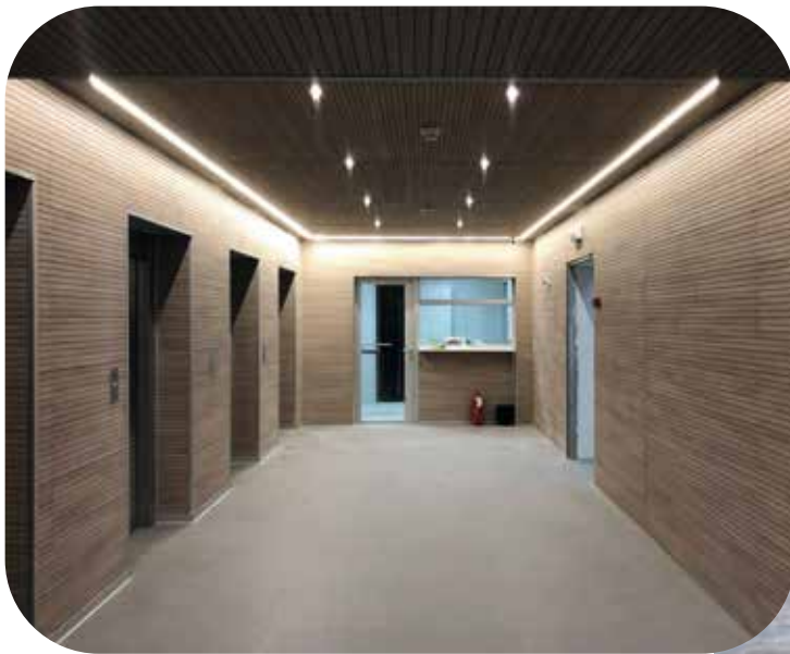
MELAMINIUM WOODENWOOD PANEL B; S2;do / WOODEN PAINTED TH. 14 MM. HOLE D.0,5 MM. PITCH 6X6 MM. BLACK SOUND-ABSORBING FABRIC IN THE BACK
